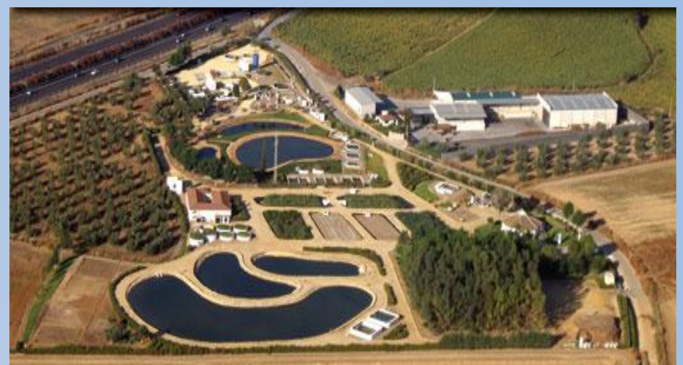
Figure 1. Experimental Plant of the Foundation Centre for New Water Technologies (CENTA) Carrión de los Céspedes (Seville)
