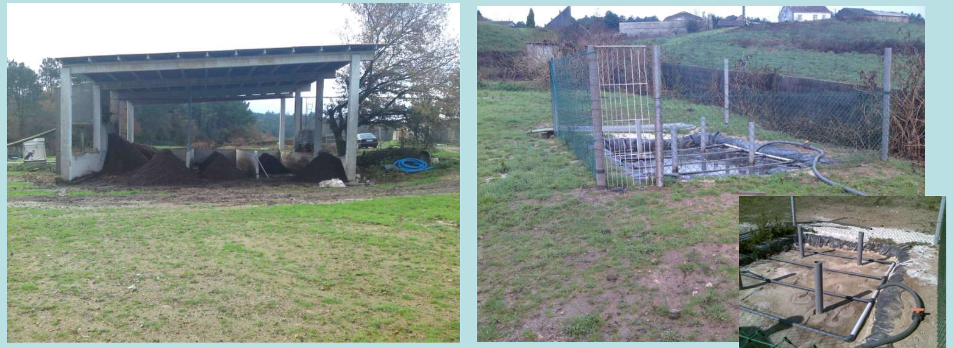
Figure 1. Composting plant (1a, left) and VFCW system (1b, right) used to treat swine manure
