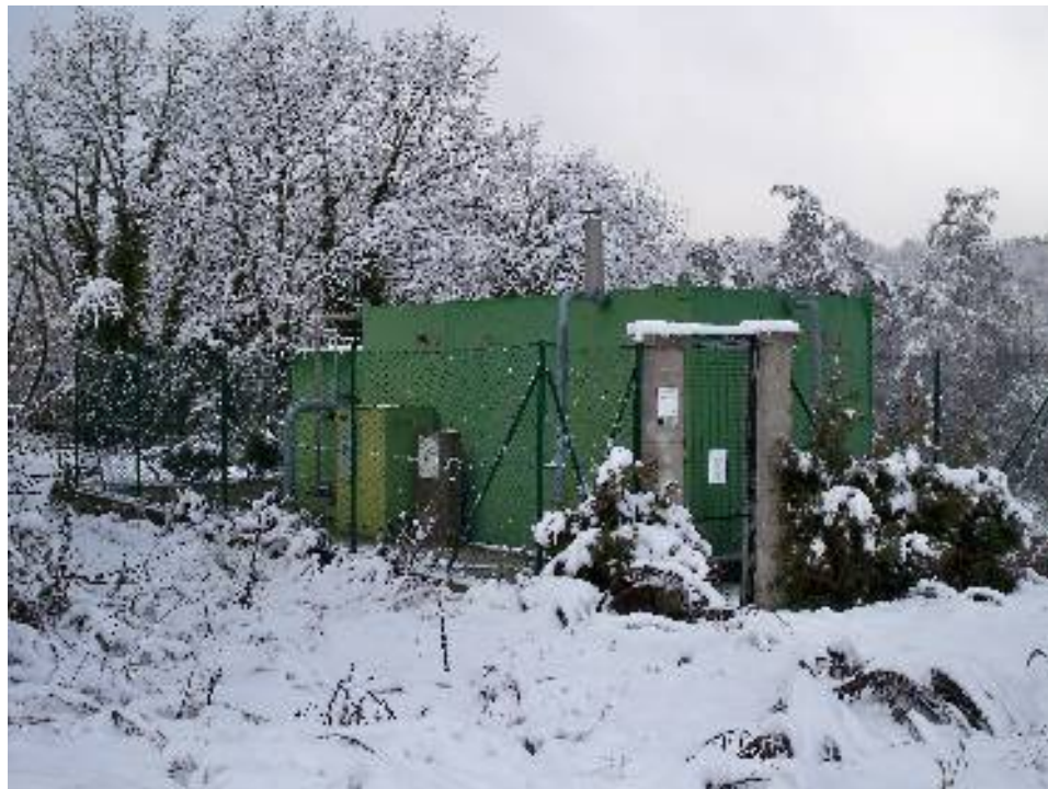
FACET STP TREATMENT PLANT
