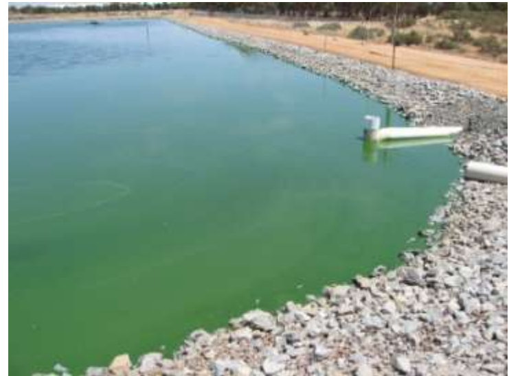
Merredin WWTP (Barrington 2009)
