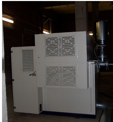
Figura 2.- Magnetic levitation turbo-compressor
