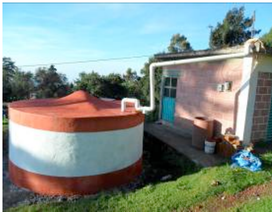
Figura 2. Rain water harvesting.
